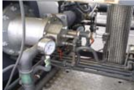
Heater burns diesel oil for operation safety
