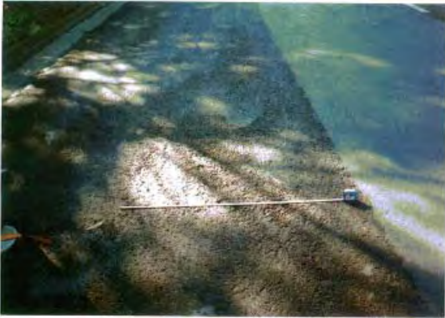
Aggregate Scattering Spots
