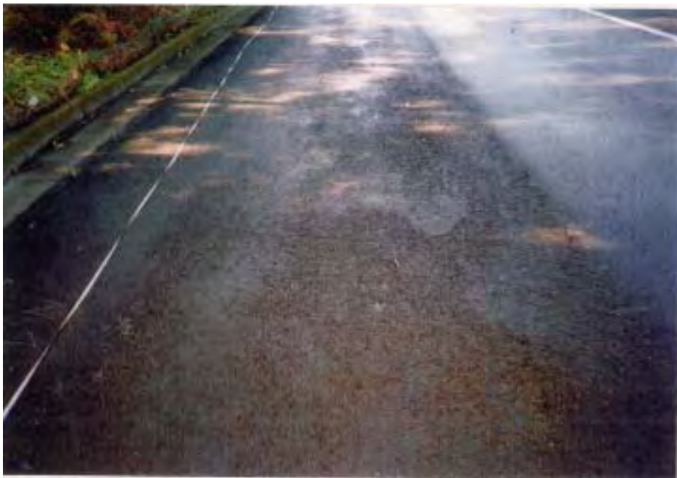
Photo-3 Aggregate scattering spots
