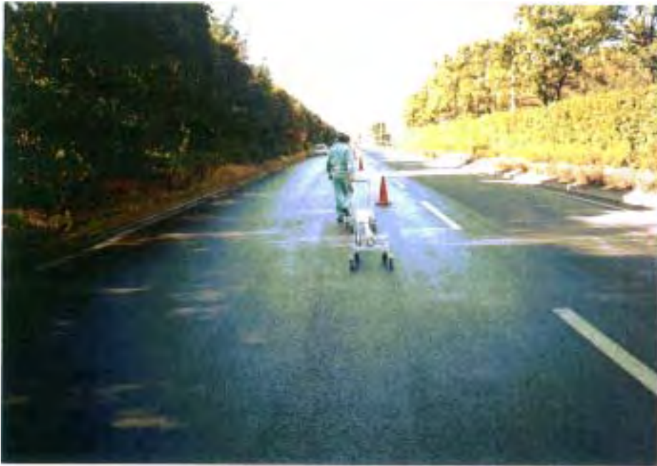
Measurement of Longitudinal Roughness
