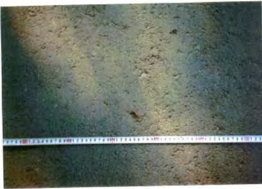
Close up of Road Surface (Job Site #1)
