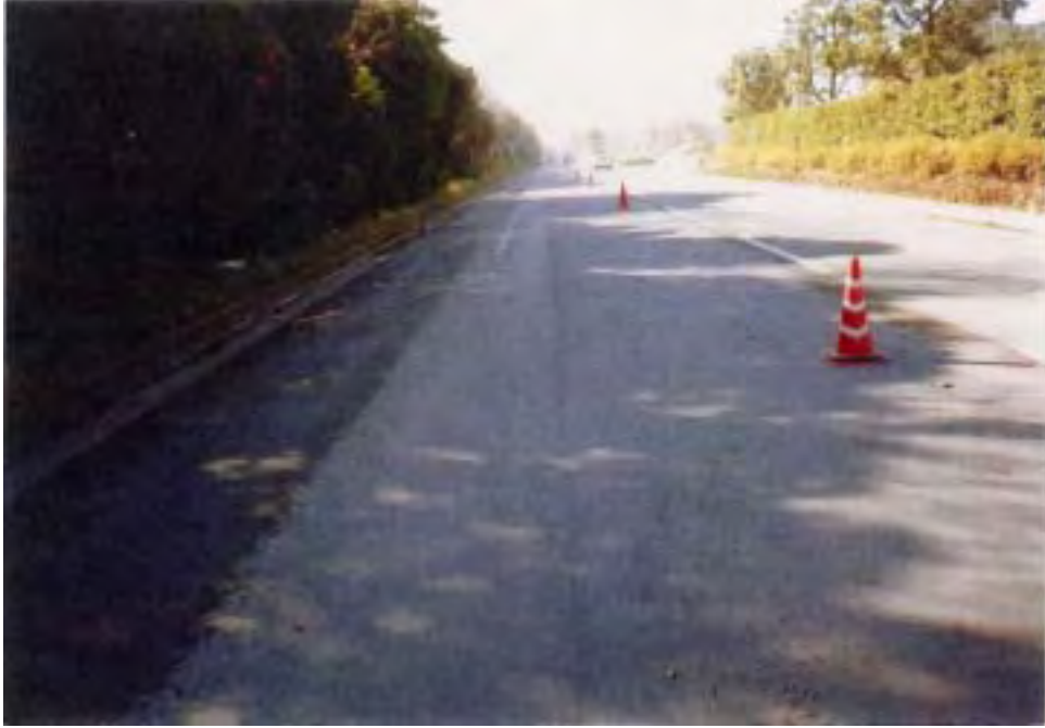
Photo-2 Job Site #2
