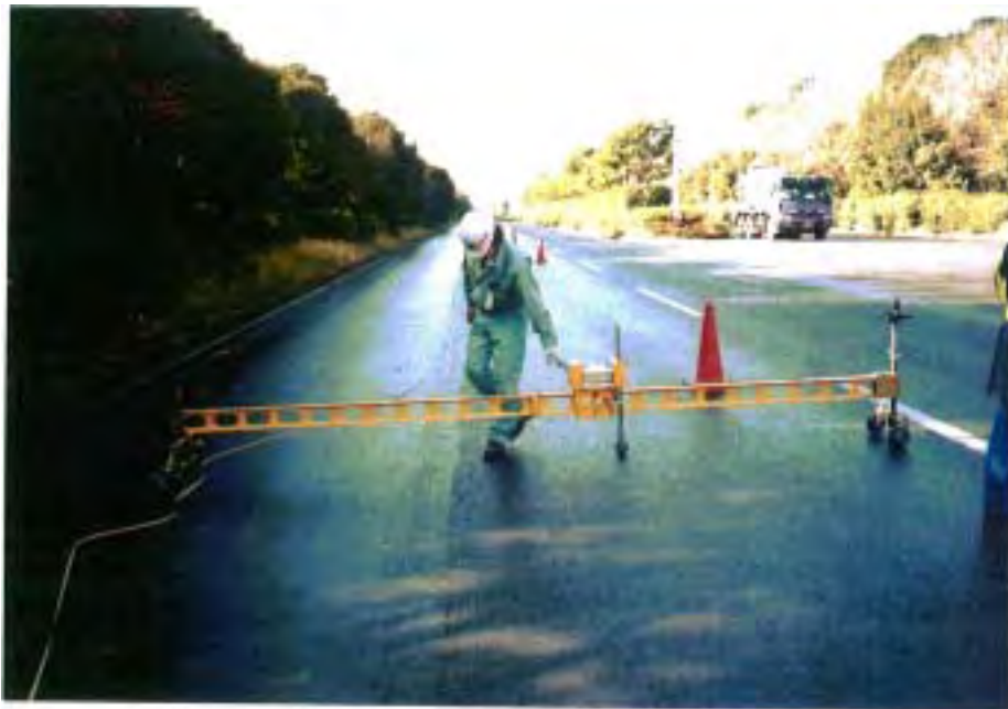
Measurement of Rutting Depth
