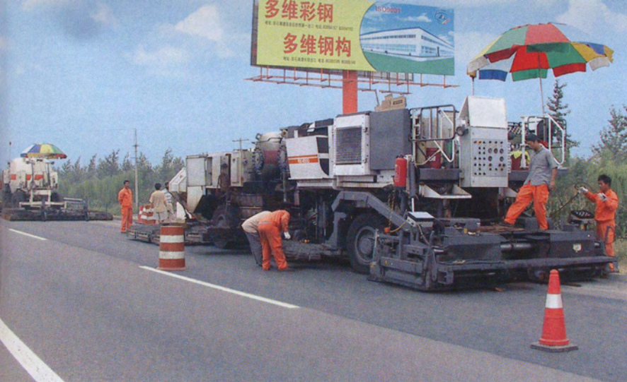
The Wirtgen train rehabilitates a section of the Jingjintang Expressway in China
