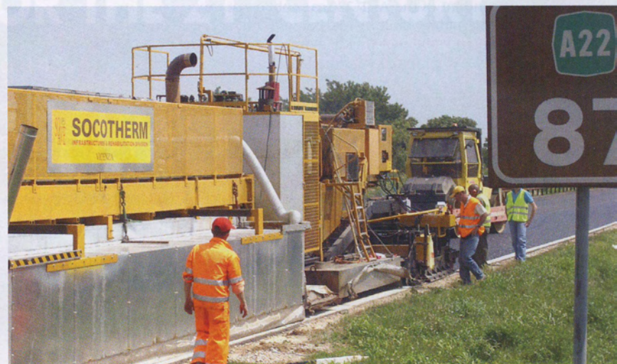
Left: A PAVIREC machine at work on A22 Highway, and right: a detail of the machine at work
