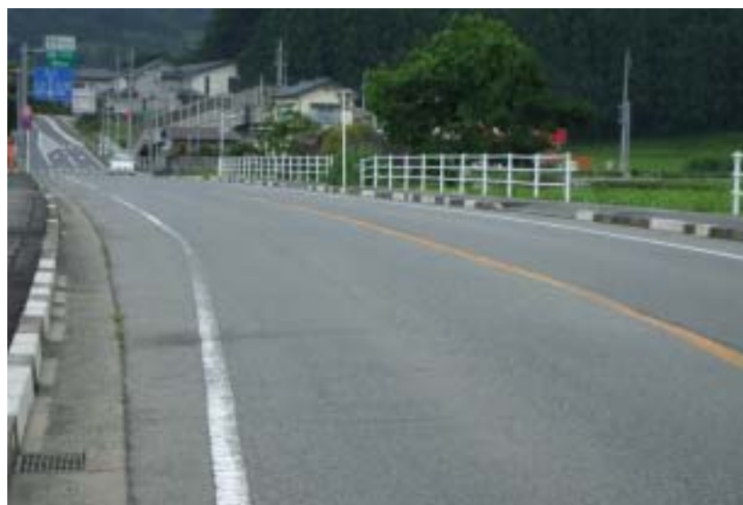
Photo1 Recycled pavement in service for 7 years (Minakami City road, Toyama prefecture, Japan, Photo taken in July, 2007)
