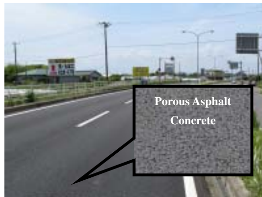
Photo3 National Road Route126 in Chiba Prefecture
